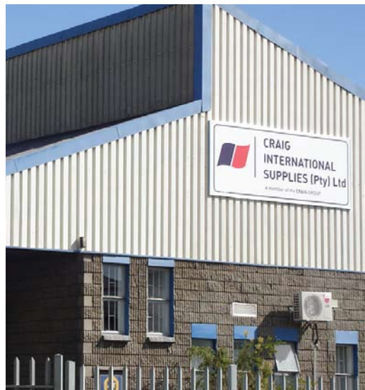
CIS Pty's new base, Cape Town.
